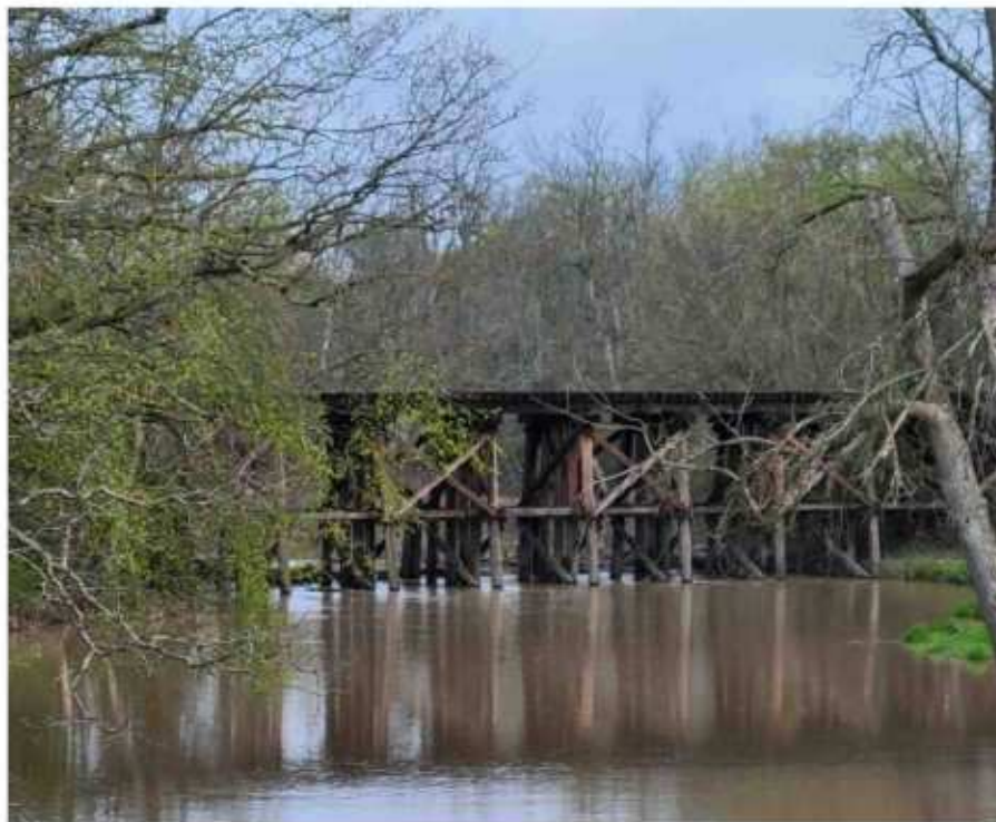
FIGURE 4.6: WOODEN TRESTLE BRIDGE
