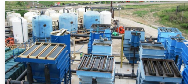
Removed Water Treated in Staging Area at Temporary Water Treatment Plant
