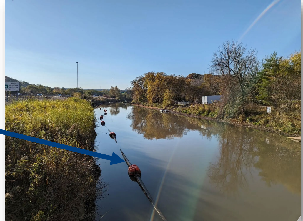
Hydraulic Dredge Pipeline Transporting Sediment to Dewatering Area
