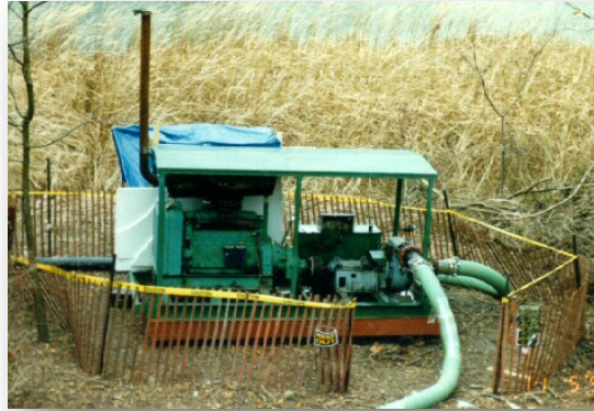
Sediment Transported to Dewatering Area through Temporary Pipeline and Pumps
