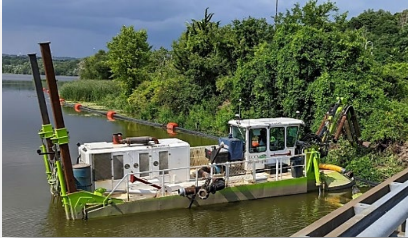
Sediment Removed by Hydraulic Dredge
