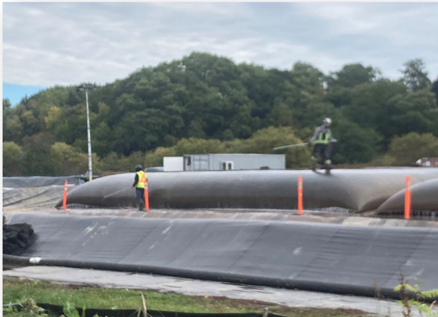
Example of large-scale sediment bag dewatering (courtesy of Canada Water Agency)
