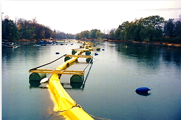
Sediment Containment Curtains
