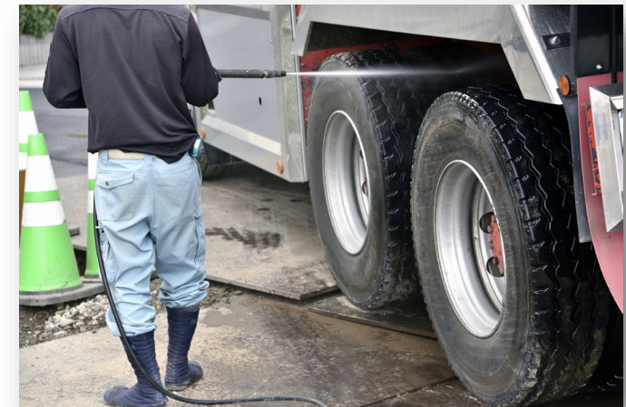
Temporary Truck/Equipment Wash Stations
