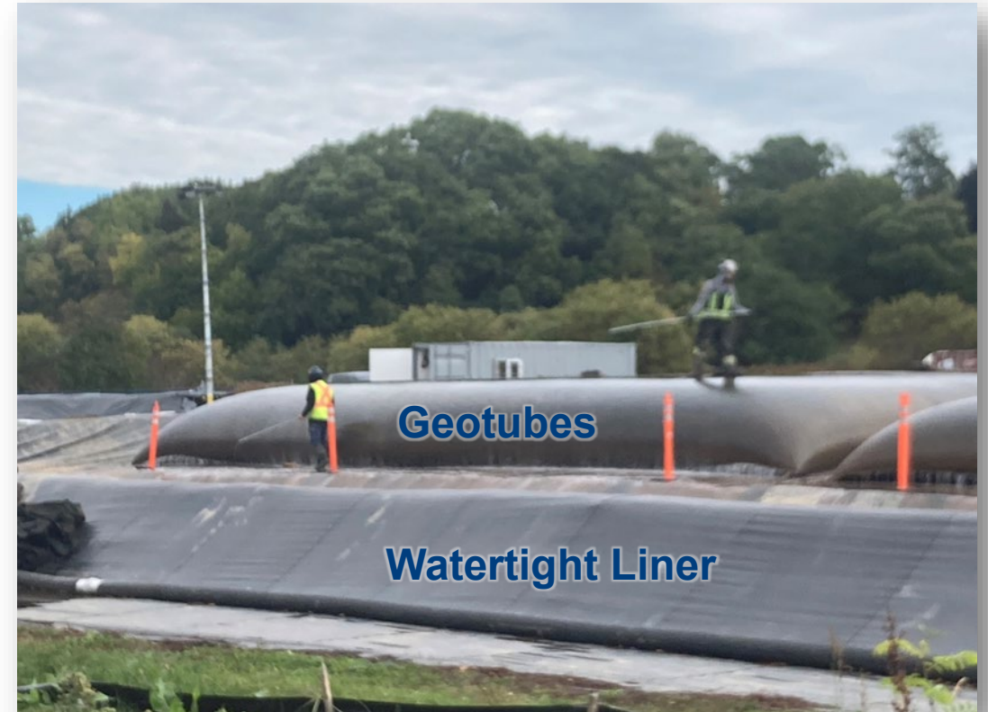
Watertight liner covers earthwork to facilitate collection of removed water and dewatering Geotubes placed inside
