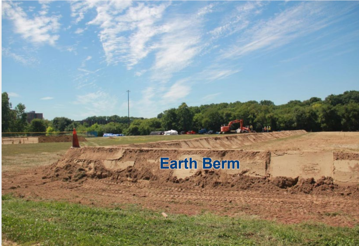
Earthwork construction of containment area
